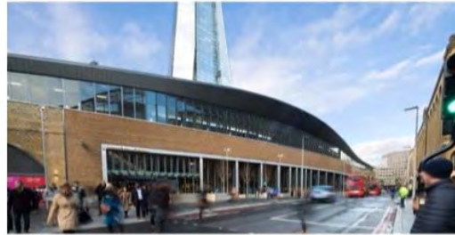
London Bridge Station
