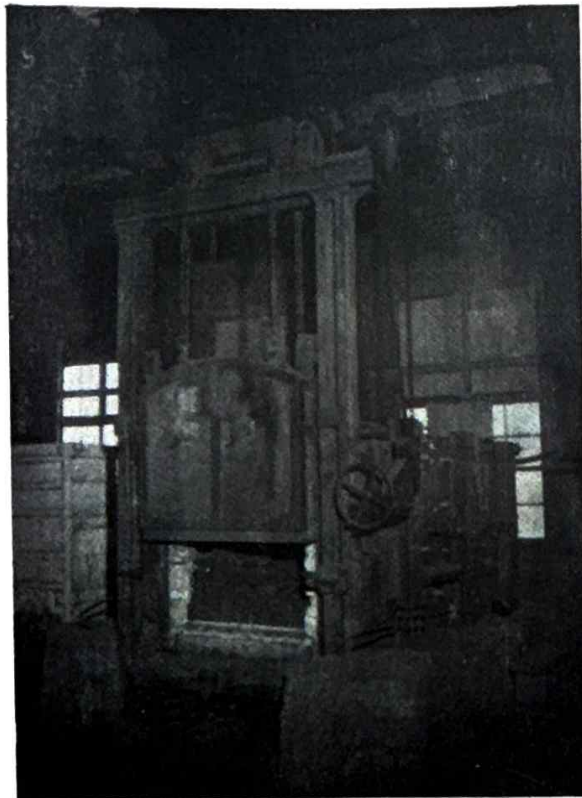
Annealing oven for rifle parts. In Building No. 12.
