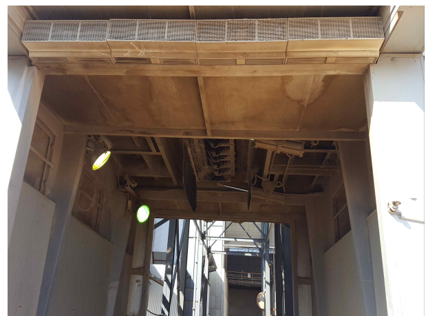
Fig. 13. The inside of the ascon hopper and the air curtain.
