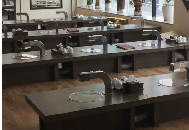
Fig. 2. Local collection for odor control in restaurants.
