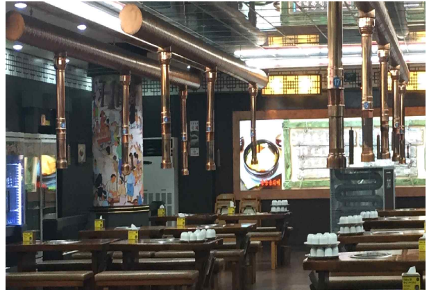
Fig. 2. Local collection for odor control in restaurants.
