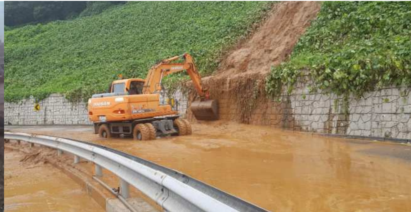
Cheonghak-dong Cheongnyang Tunnel Sediment Spill Safety Measures
