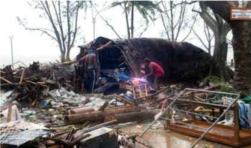
Devastation in Port Vila, Vanuatu, in the wake of Category 5 Cyclone Pam. (Photo: Alice Clements/UNICEF Pacific and Humans of Vanuatu)
