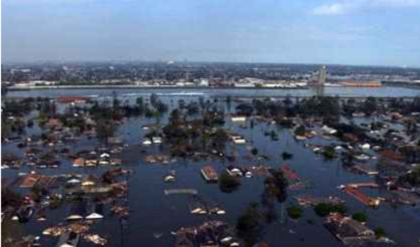
Aerial view of a flooded neighborhood in New Orleans in the aftermath of Hurricane Katrina.
