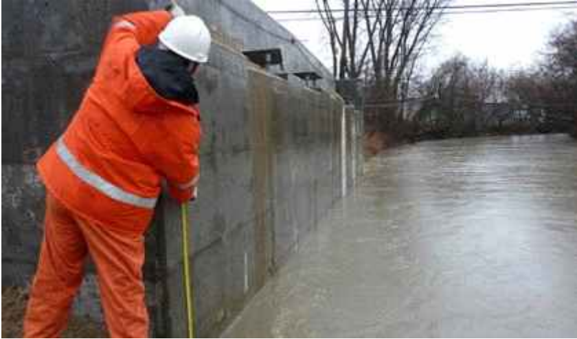
Reconstruction of a bridge after flooding. (Photo: Axel Drainville)
